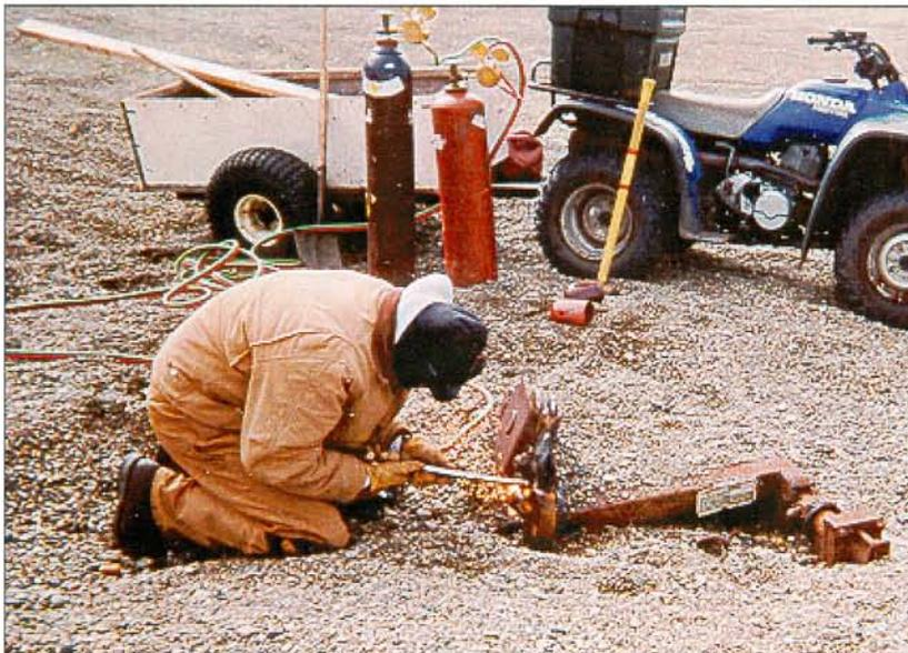
Cutting Crane Head Below the Ground Surface
