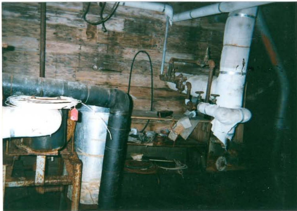
Site 18 Building 101 West - Below ground plumbing room. PACM on elbows
