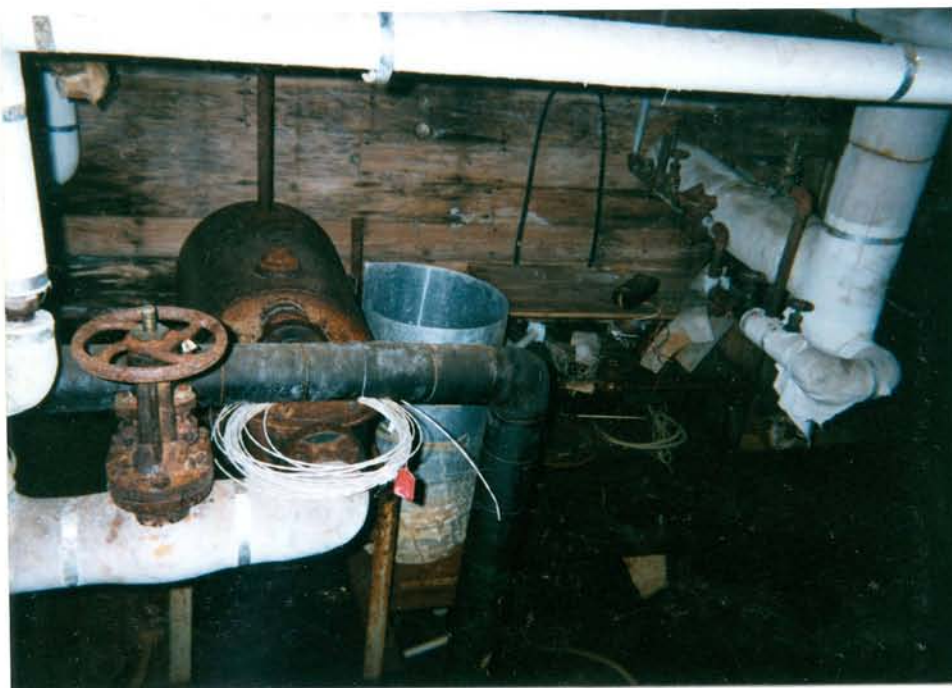
Site 18 Building 101 West: Below ground Plumbing Room, PACM on elbows.
