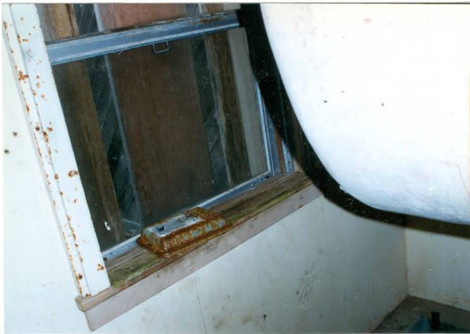
Site 18 Building 101 West: AST (500 gal.) ACM cover above opening to below ground plumbing room
