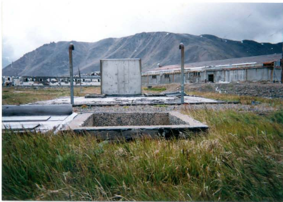
Site 21, view from Northwest. Wastewater Treatment Facility Note: 3 open Cistern Hatches and 2 vent pipes
