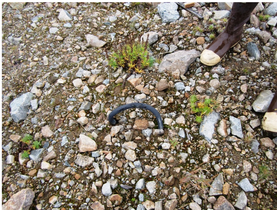
Photo No. 19 – 13 September 2013 Debris protruding through the southern side of landfill cap at Site 7.
