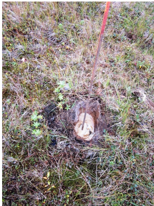
Photo No. 21 – 13 September 2013 Abandoned monitoring well filled with bentonite at Site 7.
