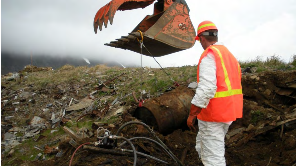
Removing pumped drum with drum lifter and excavator.
