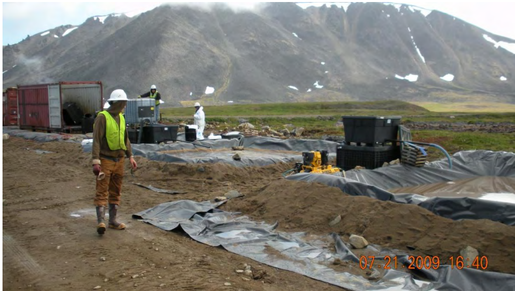
HWAP - Drum washing area with, from left to right: washing area, oil-water separating device, initial water scrubber, initial water containment, secondary scrubber, and secondary water holding area (tertiary scrubber and final holding area not shown).
