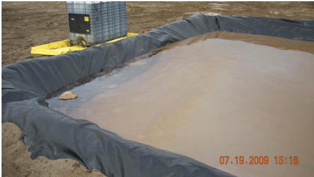
HWAP - One of the primary water containment areas with oily sheen, prior to multiple scrubbing.
