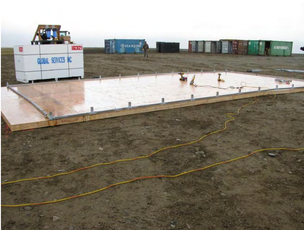
Weather port wood platform with support structure.
