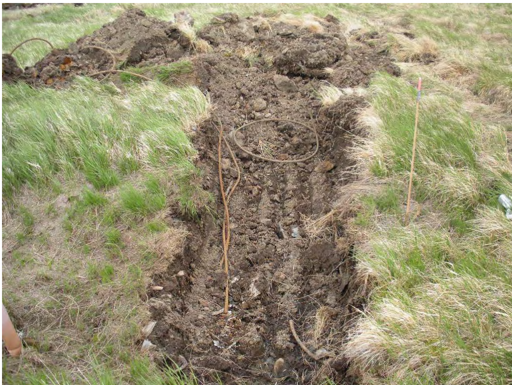
Surface area scratching in metal anomaly area, prior to drum excavation at landfill.
