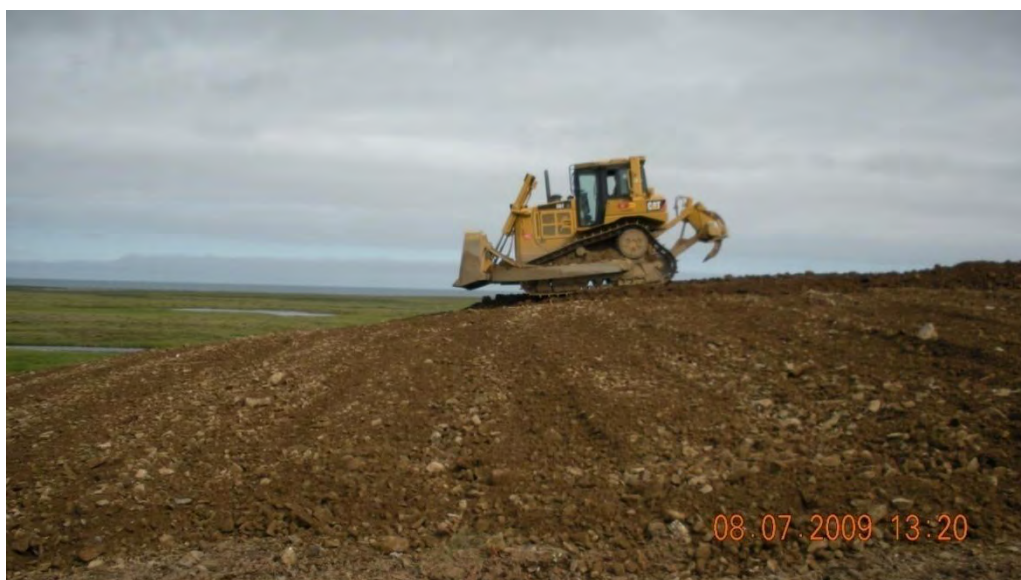
Laying down lifts for landfill cap.
