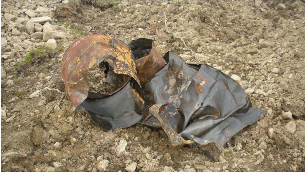
Cleaned drums placed back in landfill excavation for reburial.
