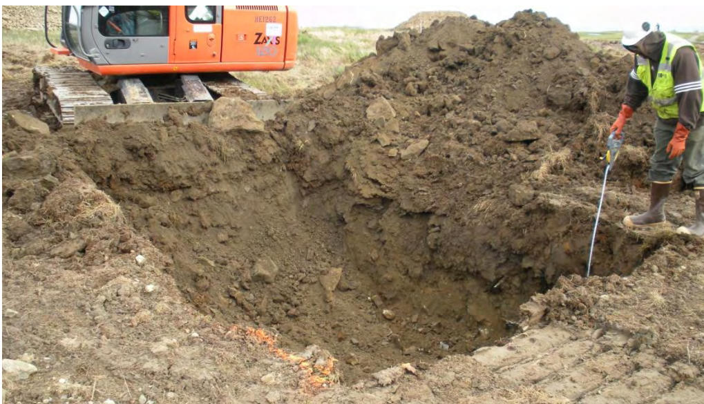
Ten-foot by ten-foot by four-foot deep investigation test pit.
