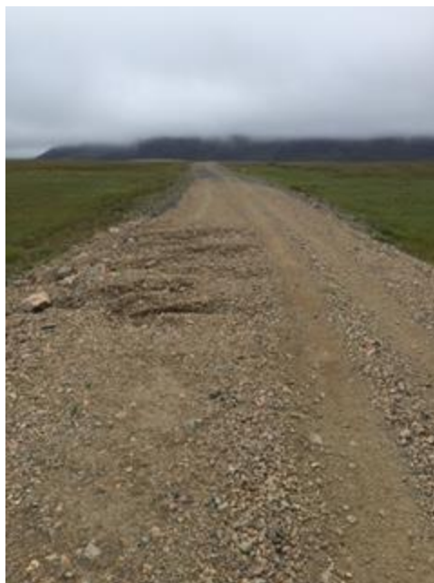
Photo No. 8 – 14 August 2016; 1245 hours. Washout near Suqi River culvert. Facing southeast.
