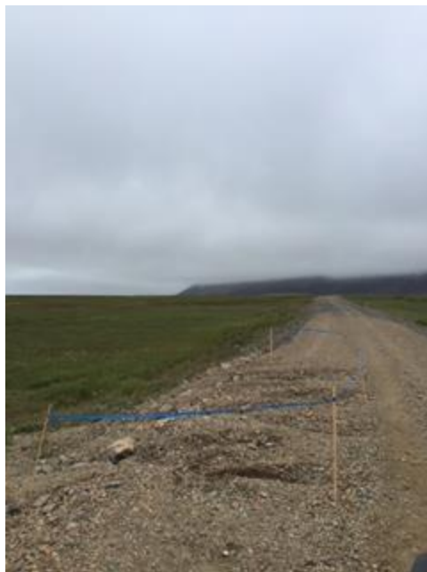
Photo No. 9 – 14 August 2016; 1253 hours. Flagging placed as safety barrier around washout near Suqi River culvert. Facing southeast.
