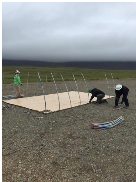
Photo No. 3 – August 2016; 1113 hours. Erecting emergency shelter. View facing south.
