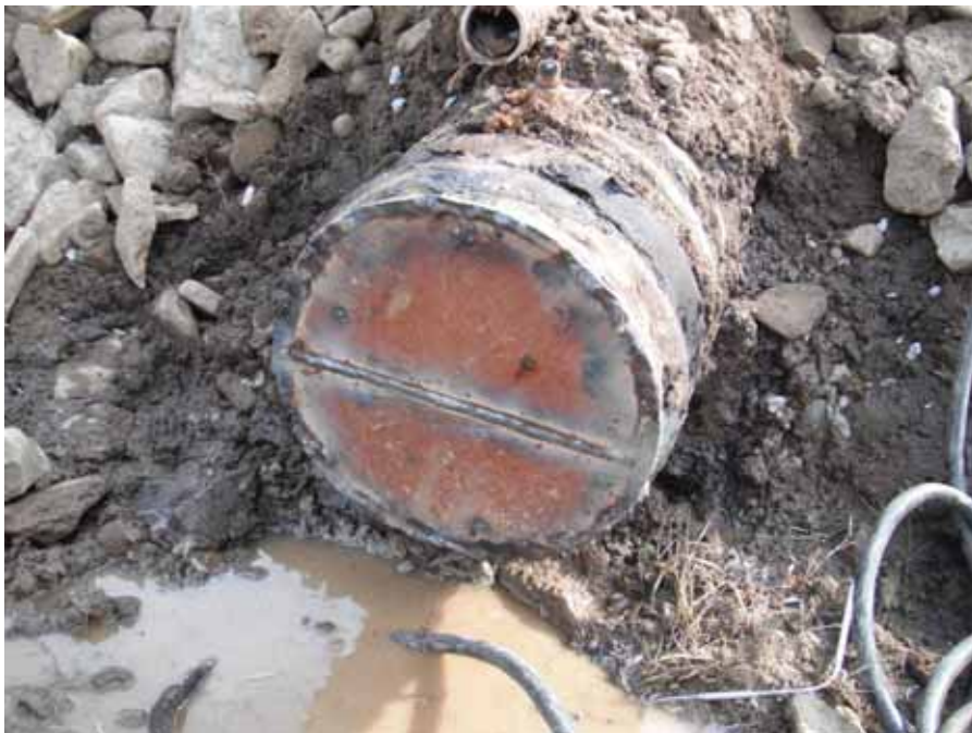
Photograph 34: Site 28 End of culvert that was detached from manhole and welded shut. Direction: downward view. Date: July 2010.
