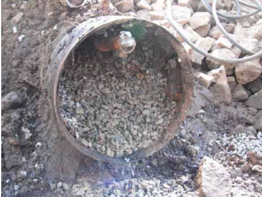
Photograph 33: Site 28 End of culvert detached from manhole that was filled with bentonite chips. Direction: downward view. Date: July 2010.
