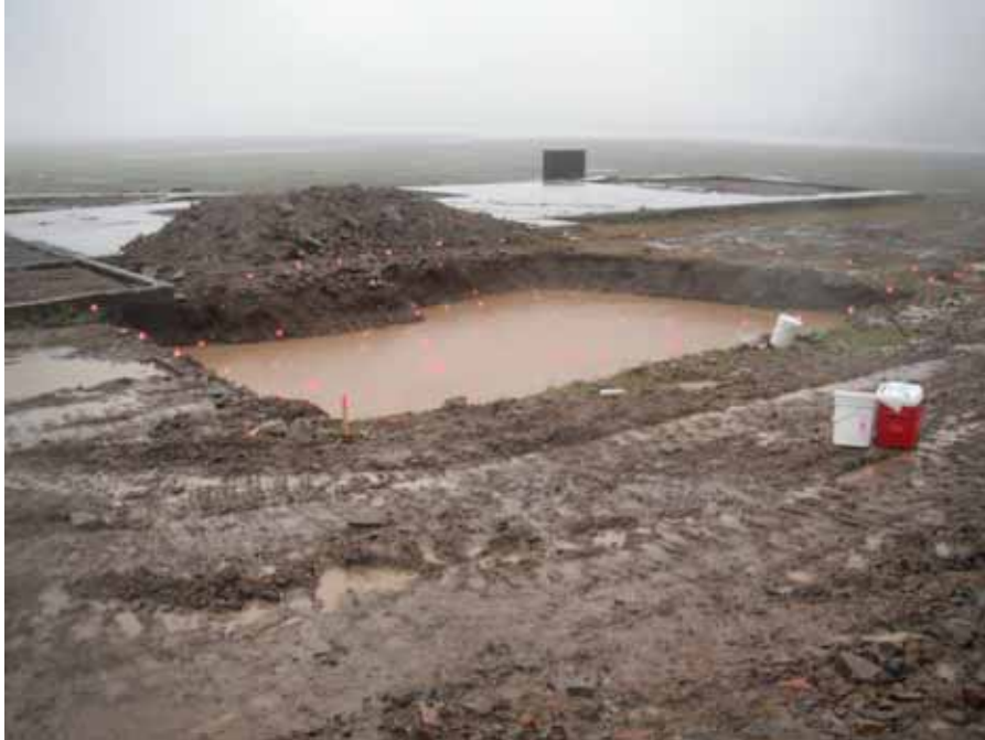
Photograph 39: Site 31 Excavation filled with groundwater and pin flags marking field-screening sample locations. Direction: northeast. Date: August 2010.
