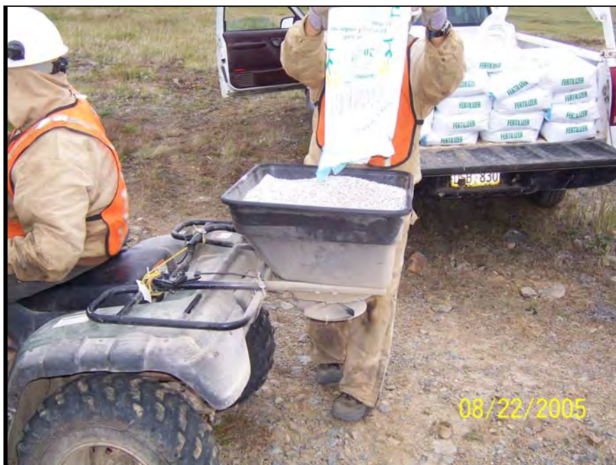
Photograph 33. Fertilizer being loaded into a spreader mounted on an ATV as part of the final seeding process around the AFS Ops Area.
