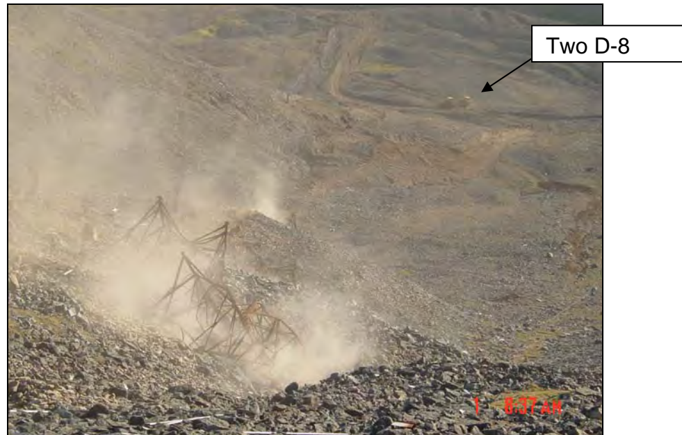
Photograph 19. After the tram tower bases were notched, two D-8 Cats were attached to the existing tram cables to pull all the tram towers down the Kinipaghulghat Mountain slopes at one time. Photo facing northeast.
