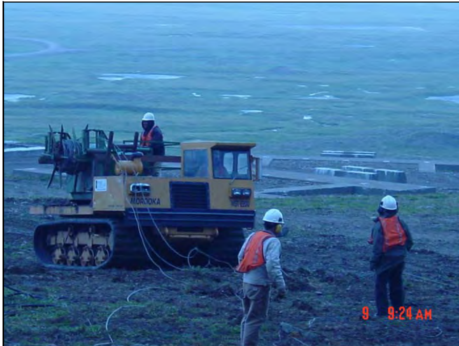
Photograph 27. Various cables and wires were spooled with a custom spooler mounted on a Morooka tracked vehicle. Note the White Alice Communications Towers footing in the background. Photo facing north.
