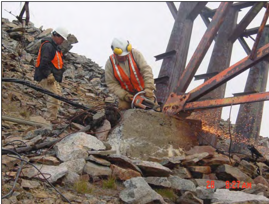
Photograph 18. BEESC crews used chop saws to notch the tram towers above their concrete footings. Photo facing north.
