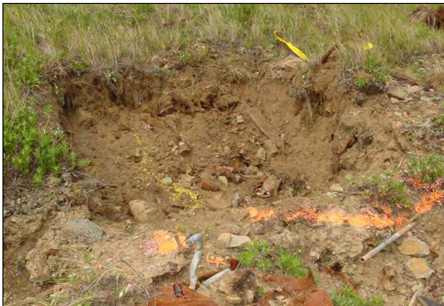
Photograph 6. CLIN 0015, Option Remove Additional PCB Contaminated Soil. Additional Soil remains at 8 locations, including Excavation 7E.
