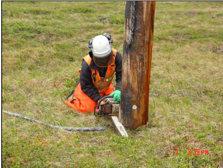
Photograph 23. Chain saws were used to cut existing wooden poles down.
