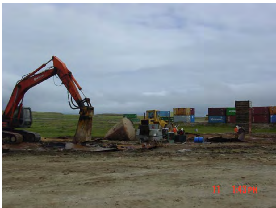
Photograph 40. BEESC nearing completion of tank scrap metal removal in the previously mentioned area. Note that all the tank scrap was removed and shipped off-island from this area. Photo facing north.
