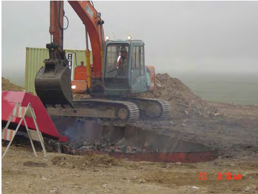
9. Lead ash being removed from burn pit and placed in Conex trailer. BEESC photograph.
