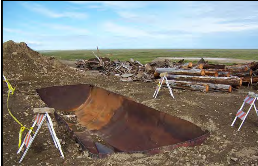
Photograph 31. Two quarters of an old AST was placed inside the 5 by 30-foot burn pit to minimize ash amounts left in the burn pit and to make removing the ash more efficient. Photo facing west.
