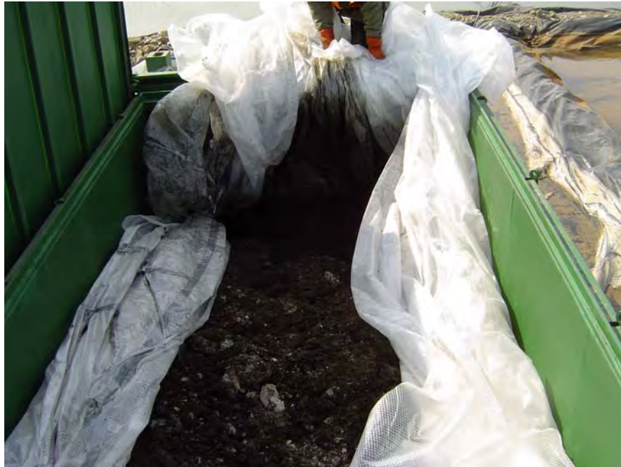
1. PCB-contaminated soil in double-lined Baker box. BEESC photograph.
