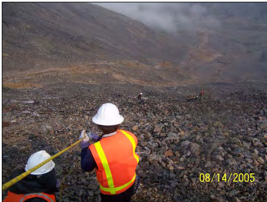
Photograph 30. A belay system was used to remove various forms for wood and metal debris from steep slopes. Photo facing north.
