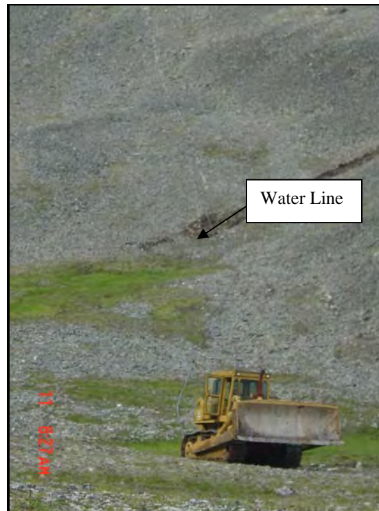
Photograph 21. D-8 Cat pulling the upper mountain complex water line down to the base of the mountain for cutting and disposal. Photo facing southwest.
