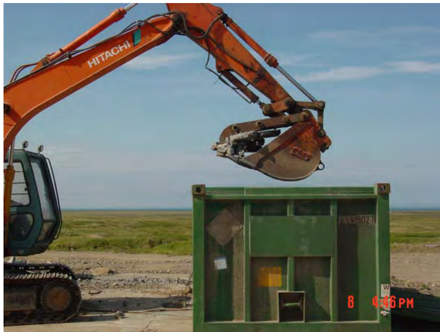
2. PCB-contaminated concrete being placed in double-lined Baker box. BEESC photograph.
