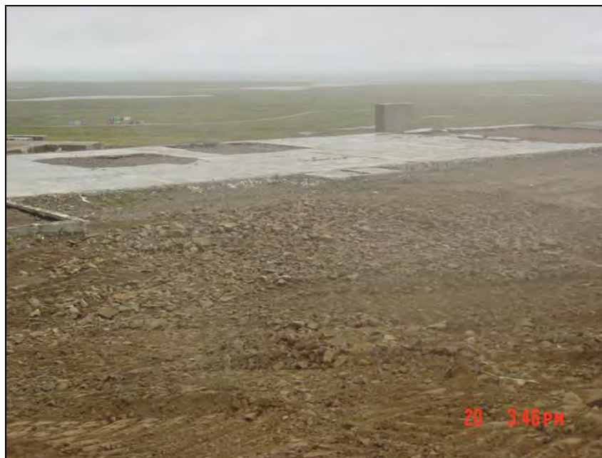
Photograph 4. CLIN 0015, Option Remove Additional PCB Contaminated Soil. Additional Soil remains at 8 locations, including Excavations 31A-1 and 31A-3. Excavations after backfilling with clean fill material.
