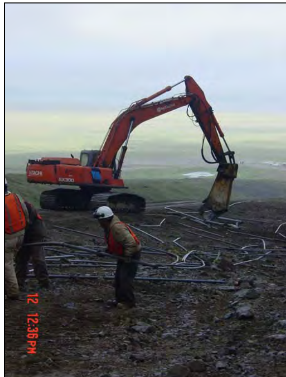
Photograph 22. Excavator outfitted with hydraulic shears was used to cut the water line. Note the BEESC crew in the foreground, placing the cut pieces of piping into a Conex. Photo facing north.
