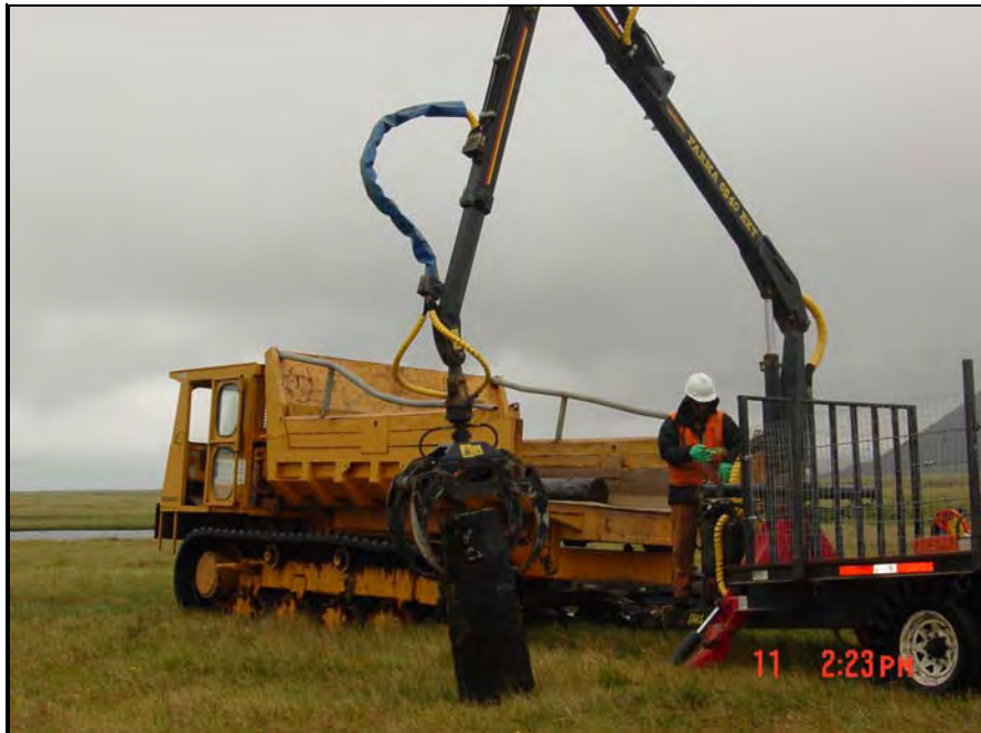
Photograph 25. A hydraulic log grapple was used to pull wooden poles out of the ground and pick up fallen poles. Note the wooden pole in the back of the Morooka track vehicle. Photo facing northeast.
