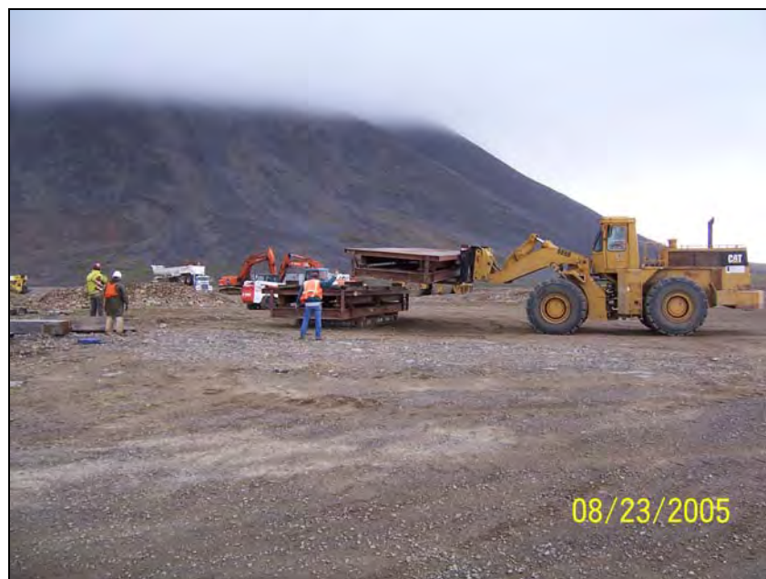
Photograph 6. Removal of the truck/waste scale during demobilization activities. Photo facing southwest.
