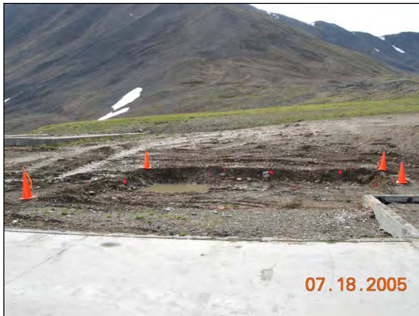
Photograph 3. CLIN 0015, Option Remove Additional PCB Contaminated Soil. Additional Soil remains at 8 locations, including Excavations 31A-1 and 31A-3. Note the standing water in Excavation 31A-3.
