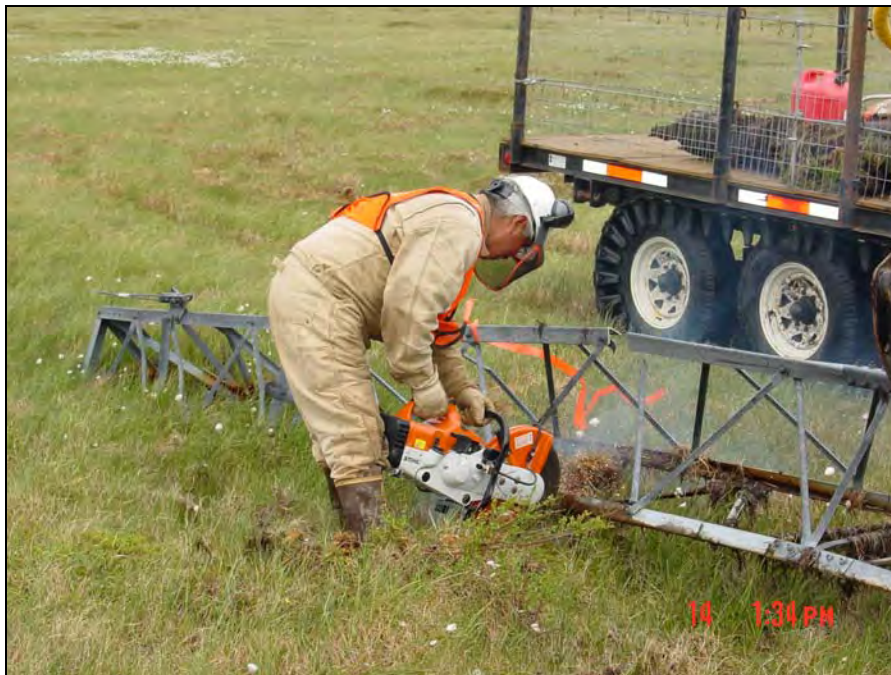
Photograph 24. Chop saws with grinder blades were used to cut existing metal poles.
