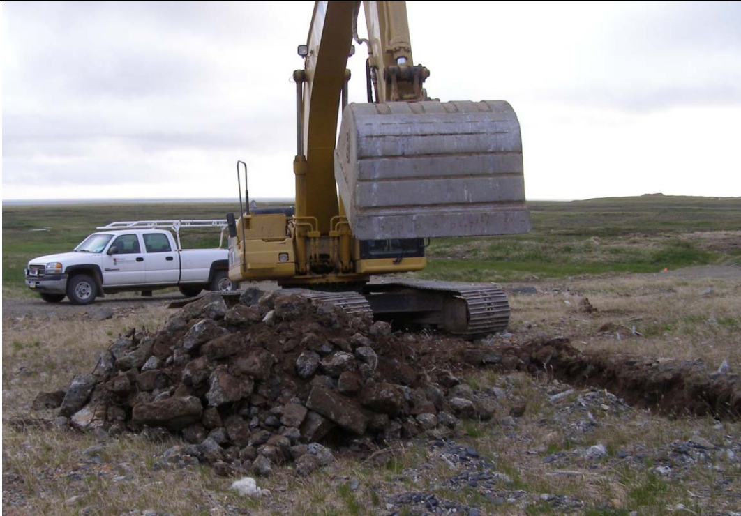
Photograph 1, July, 2009, north: Test Pit excavation, 2 cubic yard bucket.
