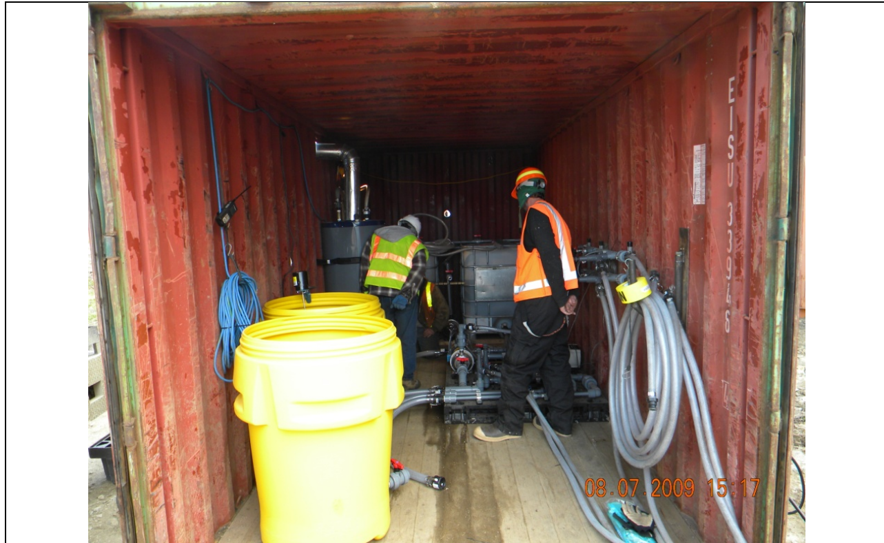
Photograph 16, 8/07/2009: View of ISCO Pilot Study Injection System Setup.
