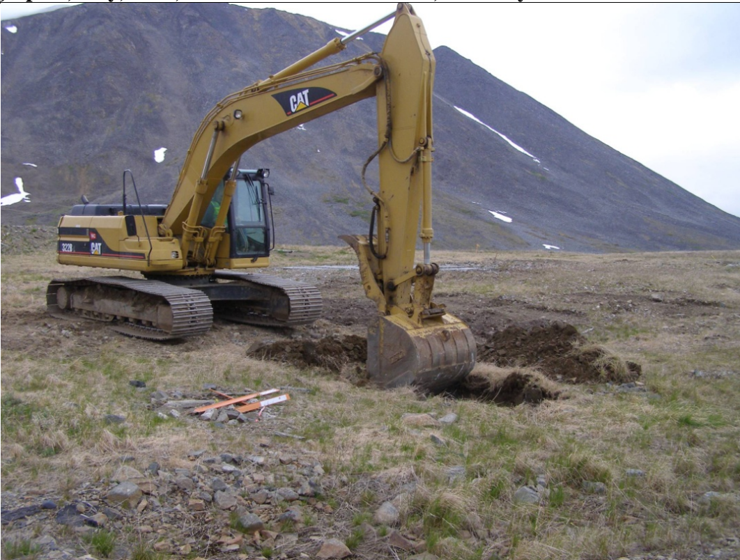
Photograph 2, July, 2009, southwest: Test Pit Excavation, CAT 322b.
