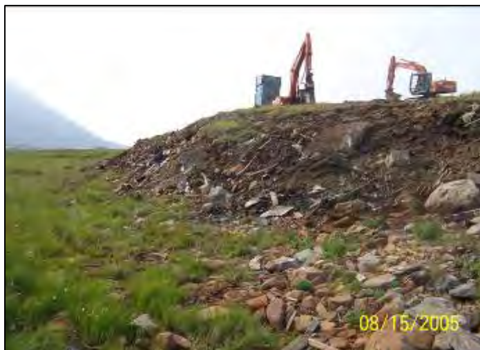
Photo (2005). View from northeast side of Site 7, looking southwest towards Cargo Beach Road (top of slope), showing completed cleanup of exposed debris on eastern edge of landfill.
