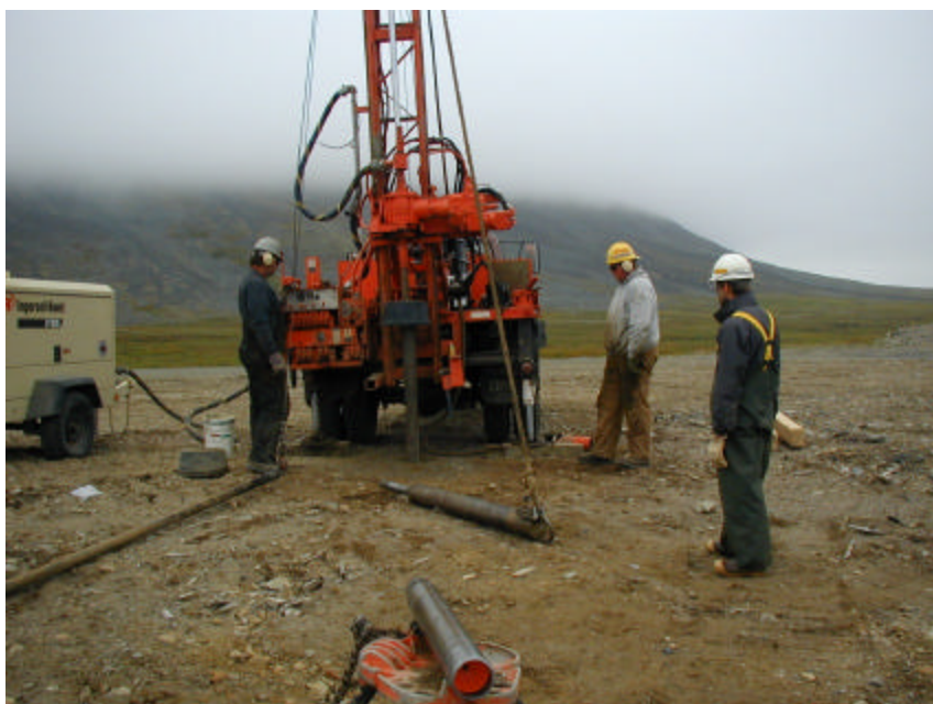
Photograph 10: Conducting the boring for installation of Monitoring Well 18MW1 using Tubex type air-rotary drilling on the regraded surface of the MOC. A cleaned split spoon sampler is in the foreground, looking southwest.
