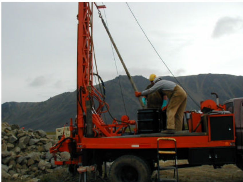
Photograph 6: Site 6 Boring 06B2 completed, decontaminating drill auger and rod in alconox solution and rinse water drums on the drill rig, looking southeast.
