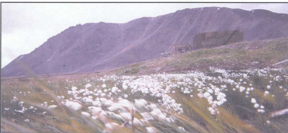
3 400,000 GAL. TANKS ON FILL PAD FROM SITE 27 HEADWATERS AREA
