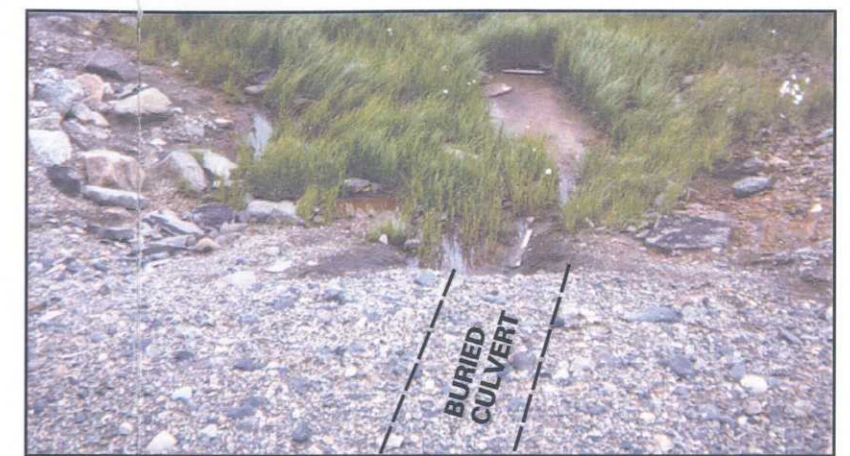
6 SITE 27 HEADWATERS AREA (CULVERT OUTLET FROM DIESEL PUMP ISLAND)
