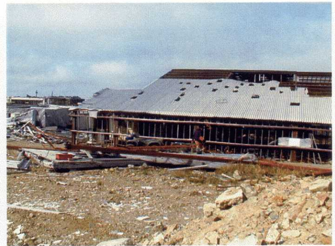
Soil Boring 22-1 and debris pile
