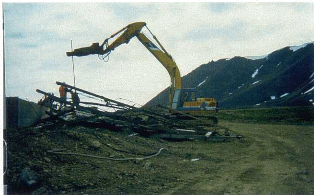
Removal of Pump from Drinking Water Well 2 01NE35GW102
