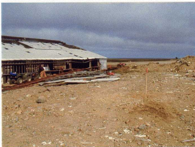
Soil Boring 22-2, 22-1 in background
