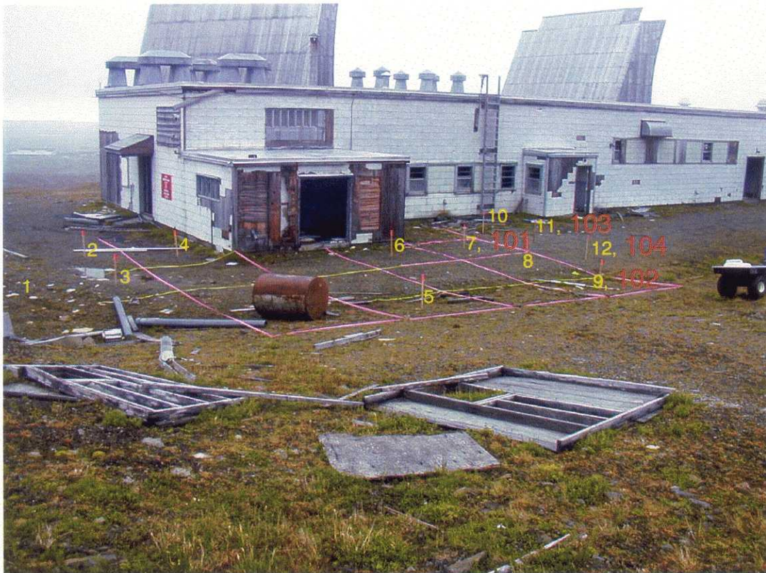
PCB Screening Grid and Sample Locations 01NE31SS101, 102, 103, 104
