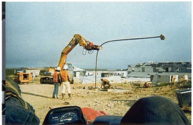
Removal of Pump from Drinking Water Well 2
