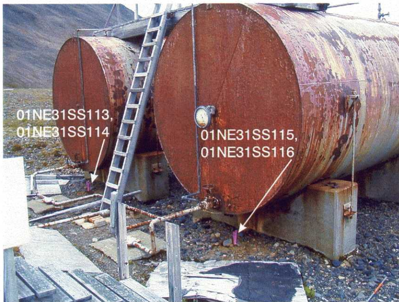
WACS Fuel Tanks Samples 01NE31SS113, 01NE31SS114 01NE31SS115, 01NE31SS116
