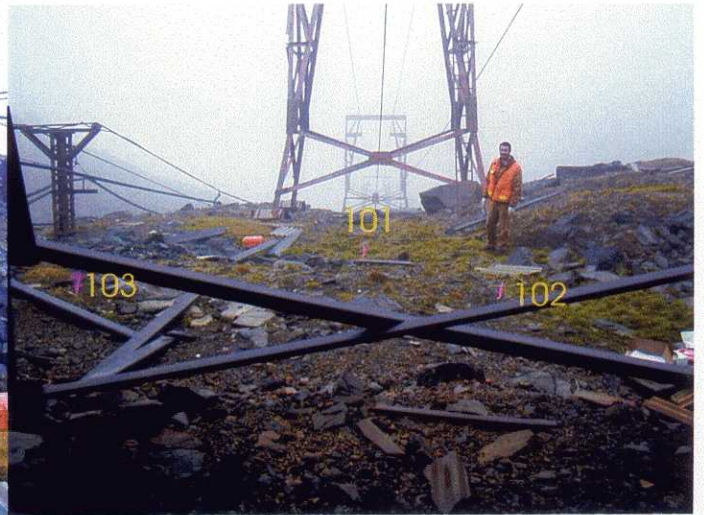
01NE35SS101, 102, 103 (Upper Tram Terminal)
