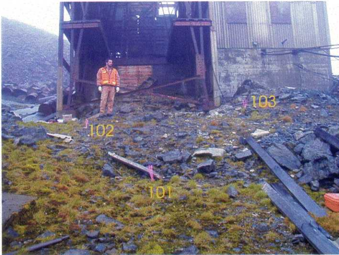
01NE35SS101, 102, 103 (Upper Tram Terminal)
