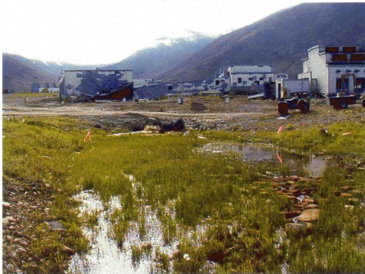
Cross Section 10 Looking South
