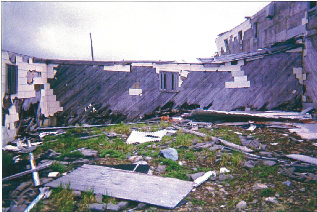
Partially collapsed arctic walkway over utilidor
