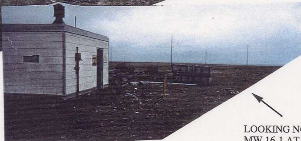
LOOKING SOUTH TANK 16-1 AT RIGHT
