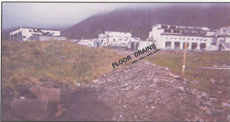
2 DRUMS AND STAINING AT SITE 13 HEADWATERS
