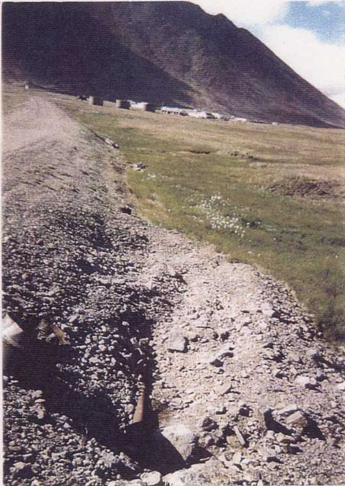
↑ LOOKING SW TOWARD MAIN COMPLEX
