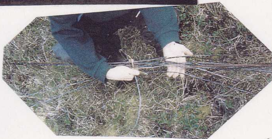
MULTI-STRAND GROUNDED COPPER WIRE
